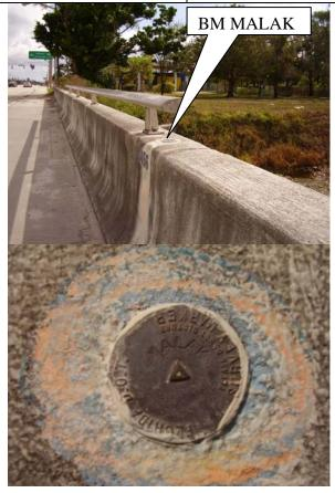
The station is a Florida Department of Transportation brass disk stamped "MALAK", set on top of a parapet Wall located on the southwest corner of the concrete bridge over the E-2 Canal on Lake Worth Road, 12.6 feet E. of the W. end of the guardrail, 8.3 feet S. of the N. edge of the sidewalk on the S. side of the bridge numbered 930456.
