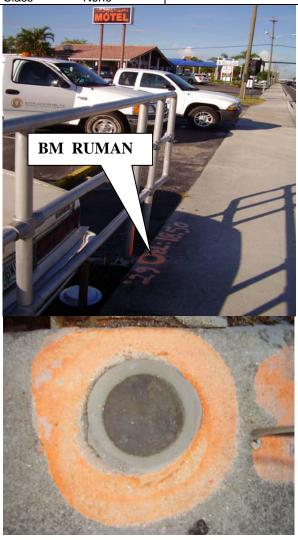
The station is a Palm Beach County brass disk stamped "RUMAN", set on top of and on the south side of a concrete sidewalk on the south side of Lake Worth Road, 0.1 mile east of Ohio Street. Also being at a catch basin which has an aluminum hand rail along the south side of the sidewalk.
