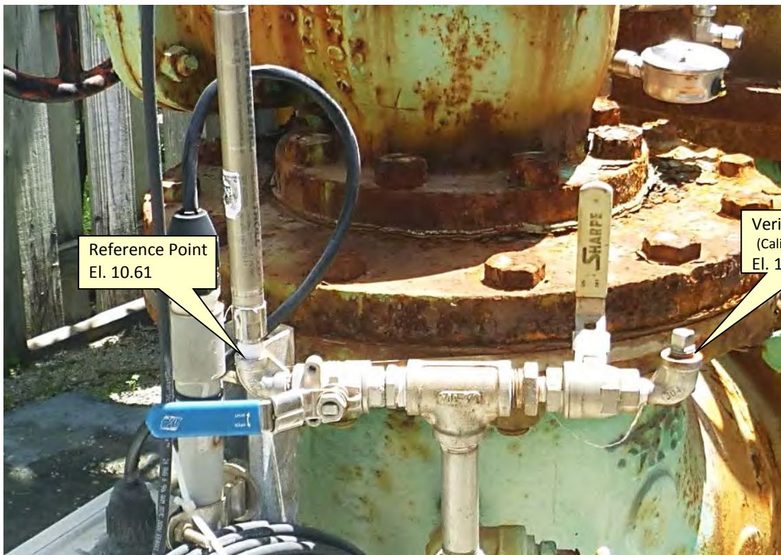
Reference and Verification Port Measuring Points
