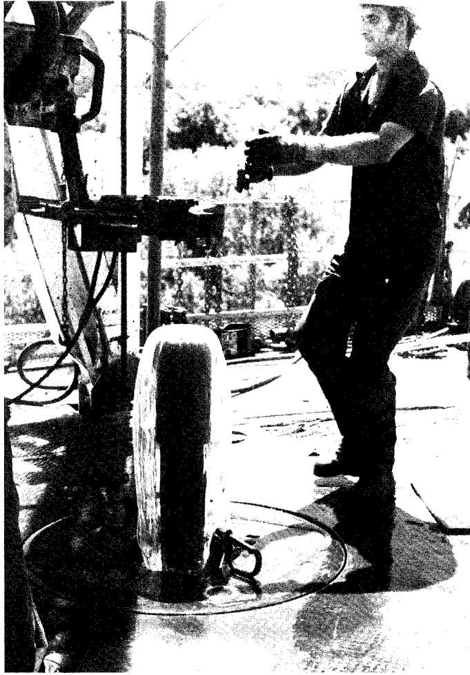
Photo 2-3. Artesian flow while adding drill pipe.
