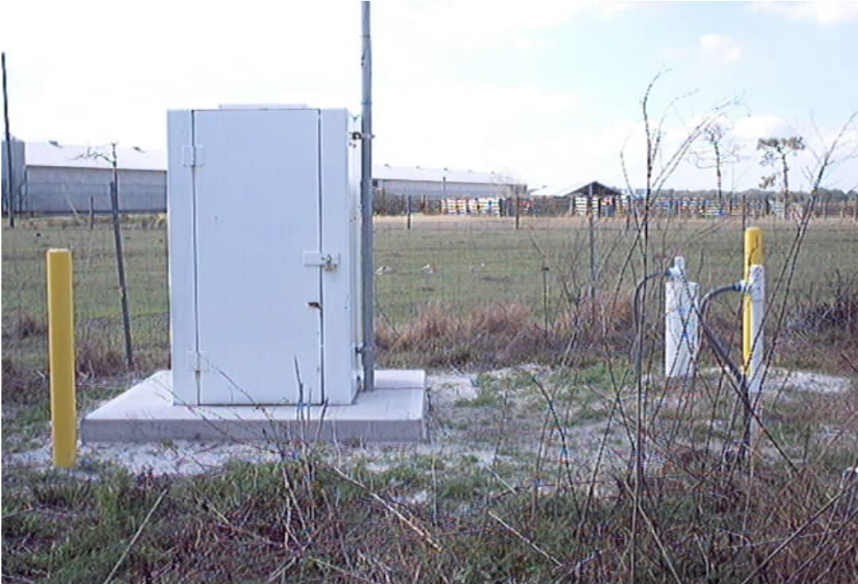
Photo 3: OSF-66, view to the northwest.
