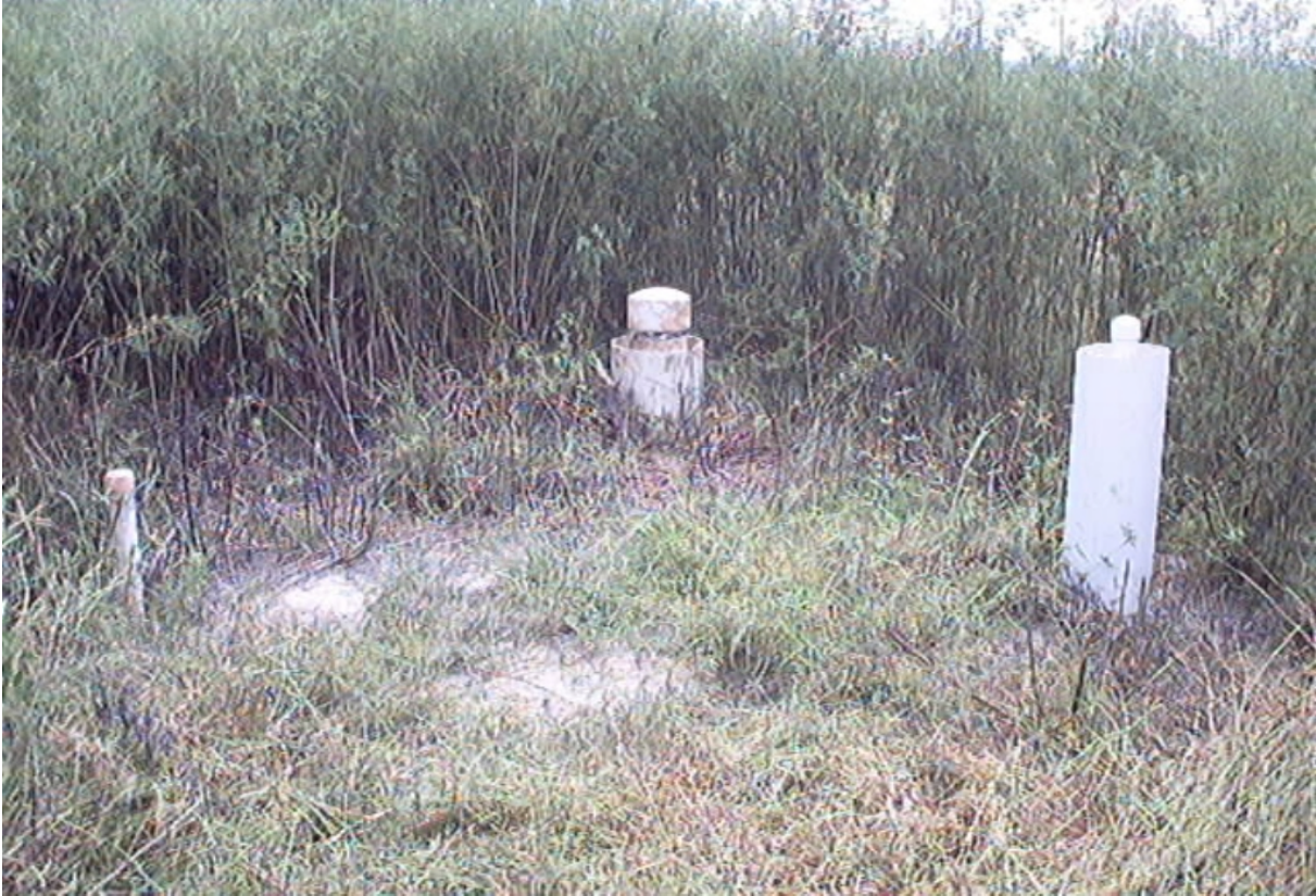
Photo 1: OSS66S, OSF-66, OSS66D before automation.
