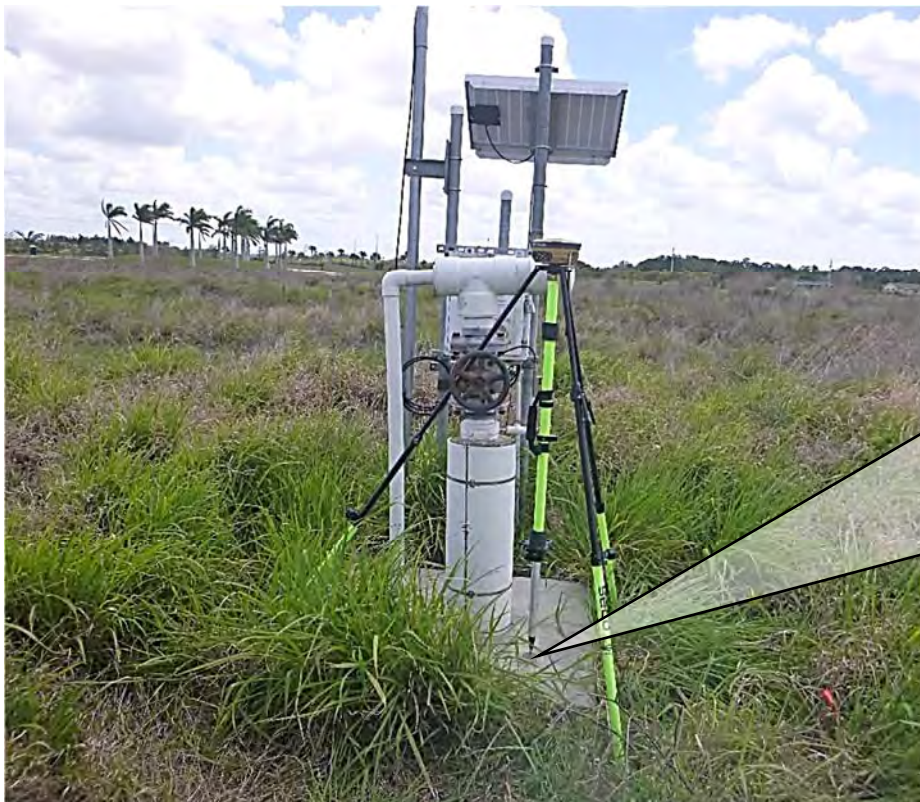
Overall Site (Looking Southerly) (27-apr-17)
