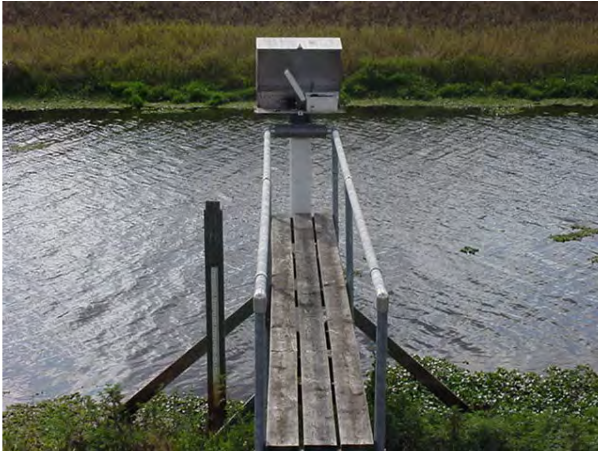
Pickett & Associates, Inc. Date of Survey: February 19, 2003 Looking: West
