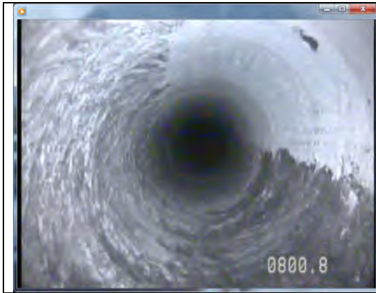
Depth: 800.8 Down view.
