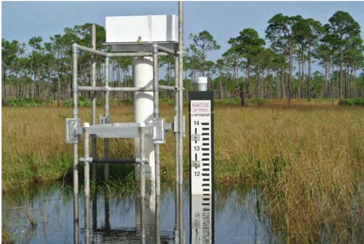
Staff Gauge (Front View)
