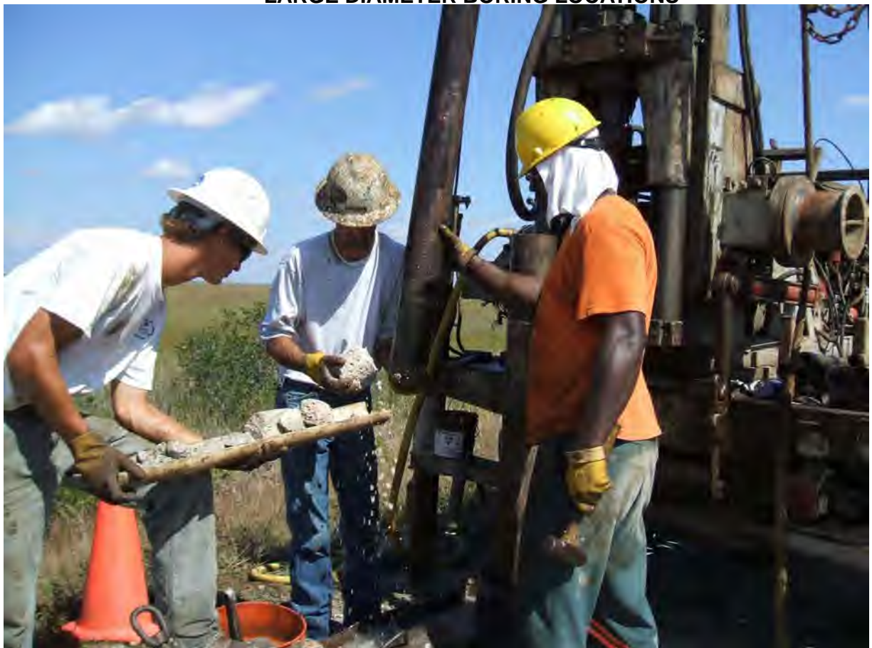
4" WIRELINE CORING SYSTEM USED TO SAMPLE TO ROCK
