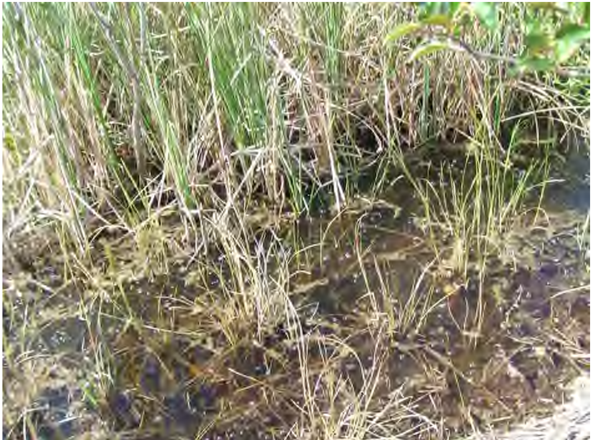
AIR BUBBLES WERE NOTED TO BE PRESENT ON BOTH SIDES OF THE LEVEE UP TO 105 FT. FROM BOREHOLES 10 MINUTES AFTER COMPRESSOR SHUTDOWN
