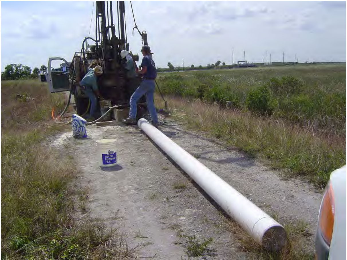
8" SURFACE PVC CASING WAS SET AT EACH OF THE LARGE DIAMETER BORING LOCATIONS
