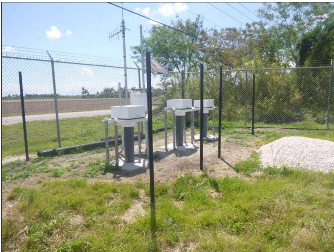
Figure 7. Completed wells with telemetry equipment installed at site P-2 (L31NW02).
