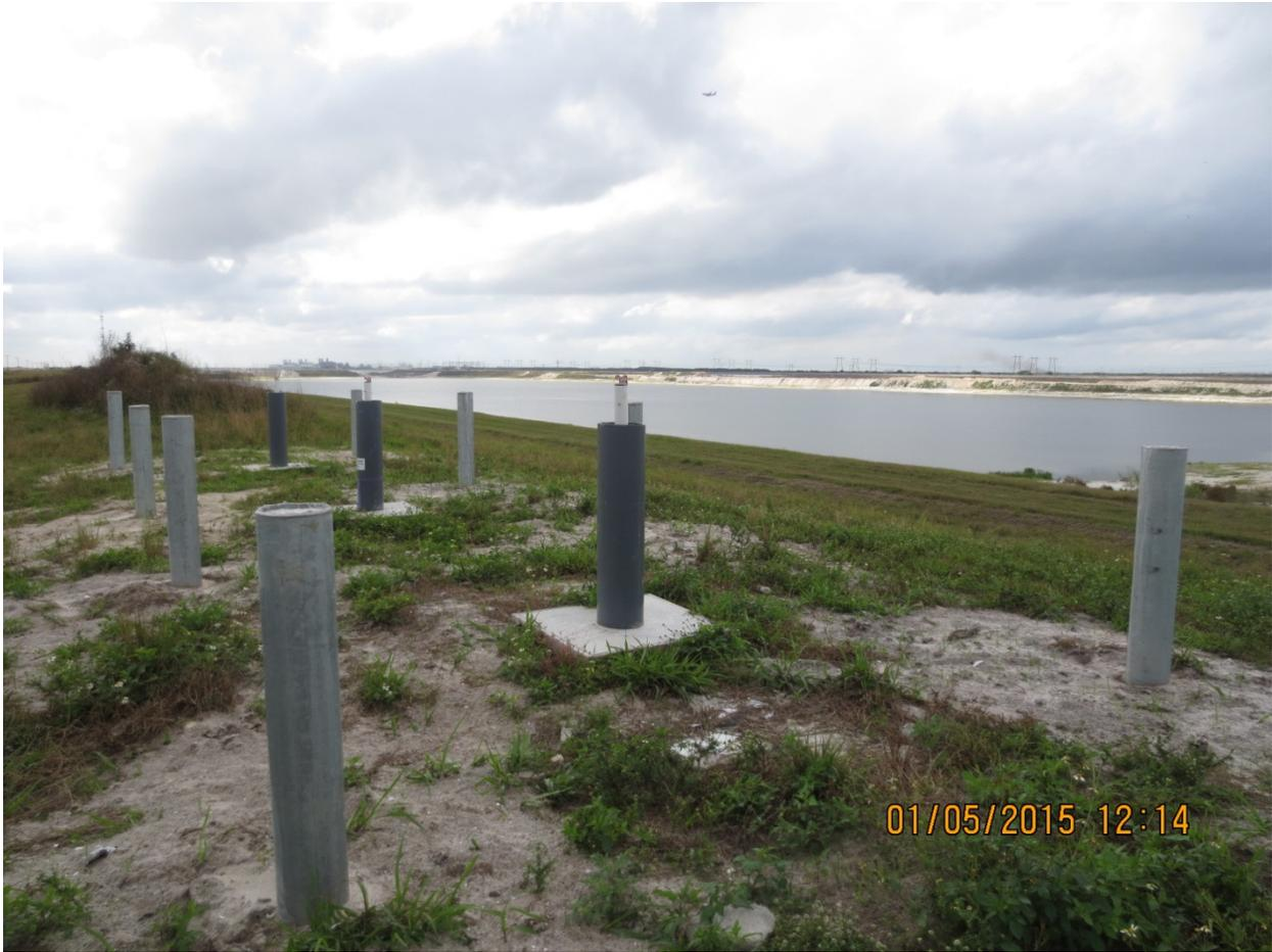
Figure 4. Photograph of Similar Well Completions (with Protective Bollards)
