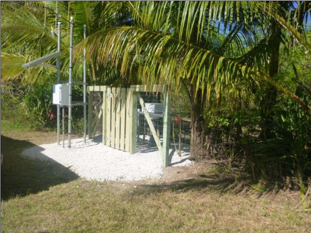
Figure 9. Completed well with telemetry equipment installed at site P-6 (L31NW06).
