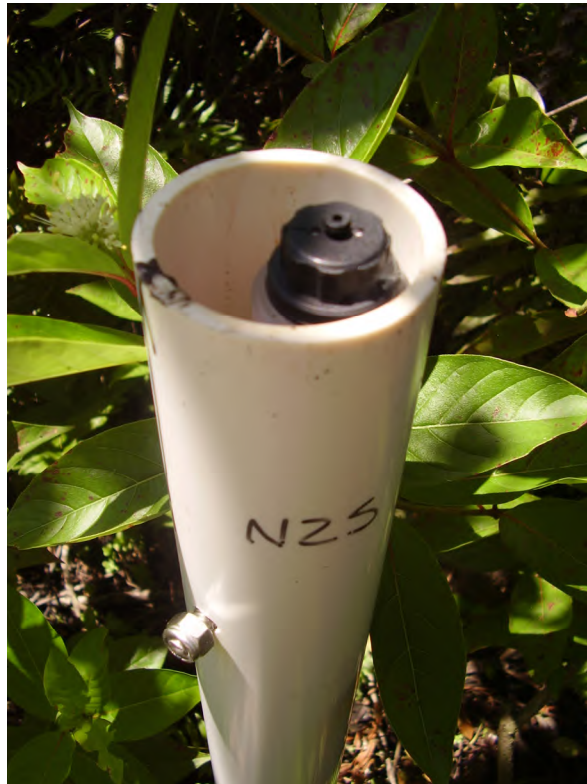
Figure 21: FIU well N2S
