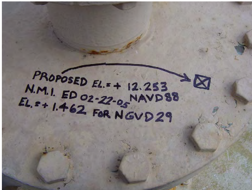
Nick Miller, Inc. Date of Photo: January 18, 2005 View: Close-up of the injection well #1 showing the contractor's markings on upper flange of T-pipe
