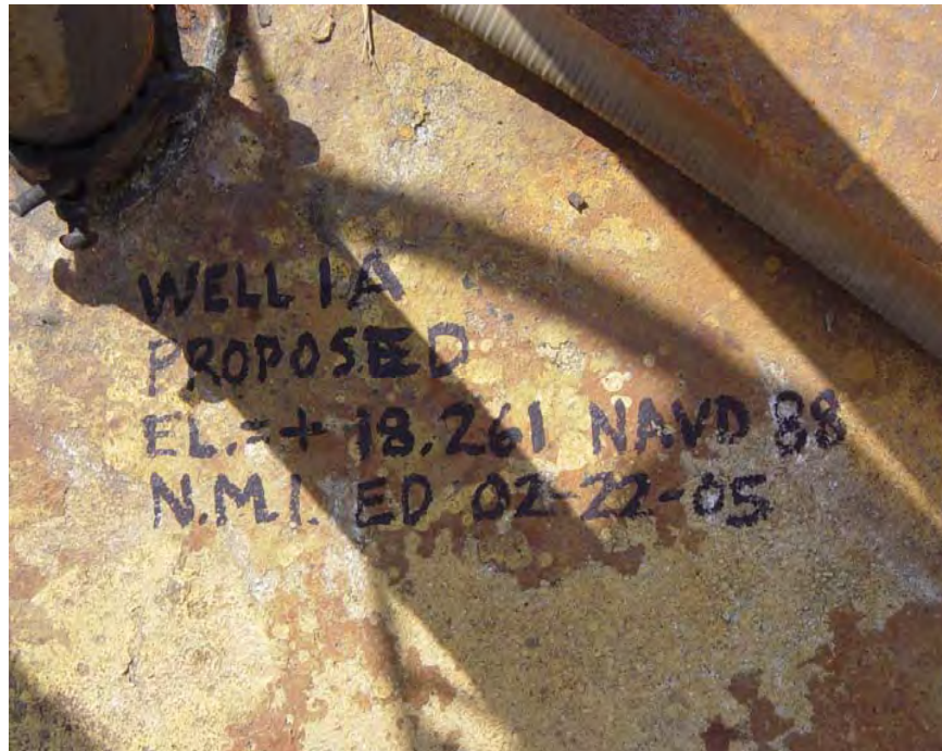
Nick Miller, Inc. Date of Photo: January 18, 2005 View: Close-up of the well 1A showing the contractor's markings
