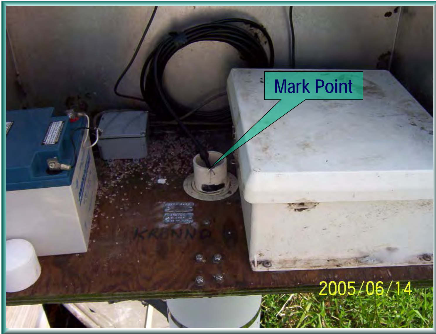
Photo Date: June 14, 2005 View: Opened well box, KRBNND.
