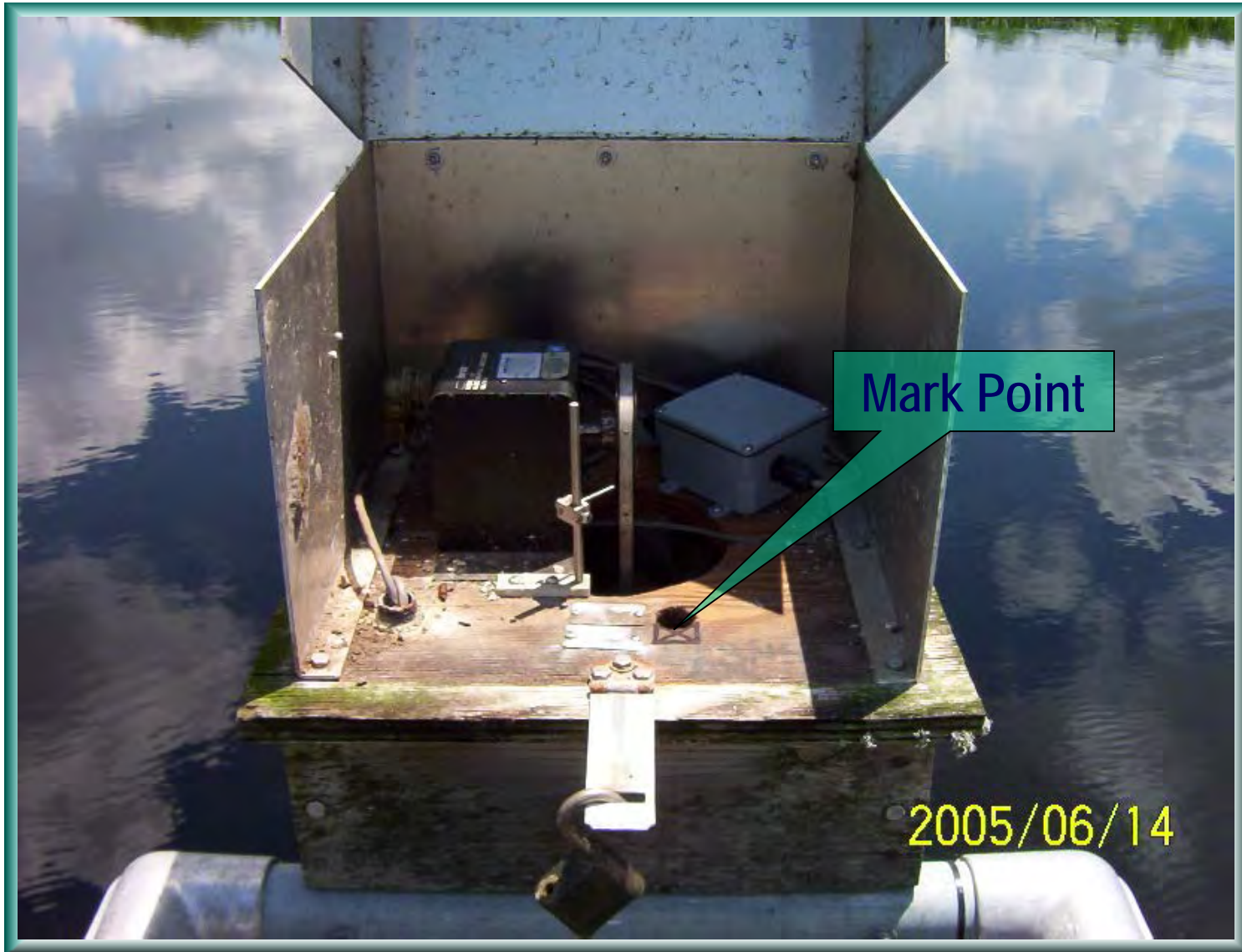
Photo Date: June 14, 2005 View: Opened well box, KRBNS.
