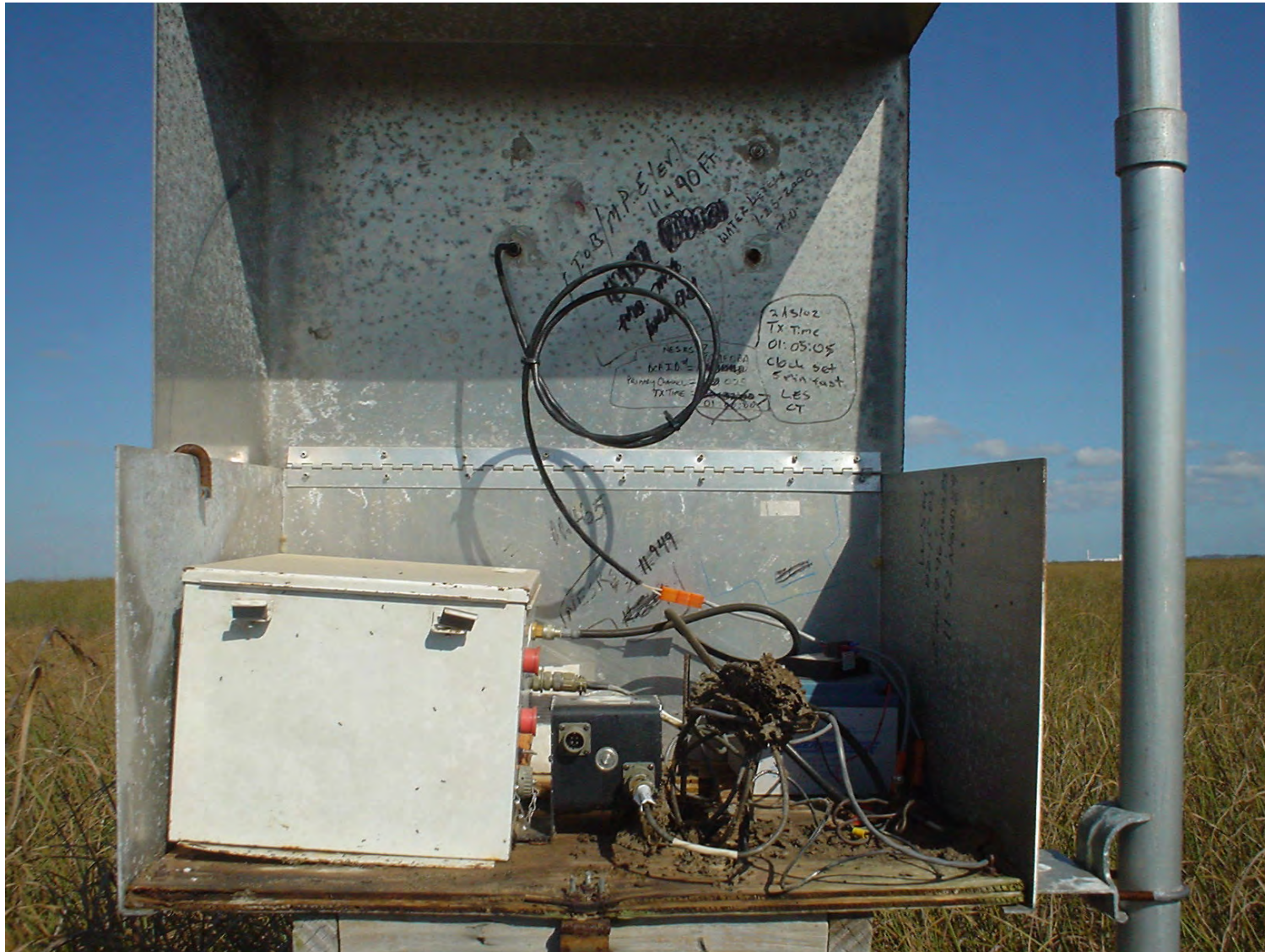
Weidener Surveying & Mapping, P.A. Date of Photo: February 15, 2005 View: Encoder Unit
