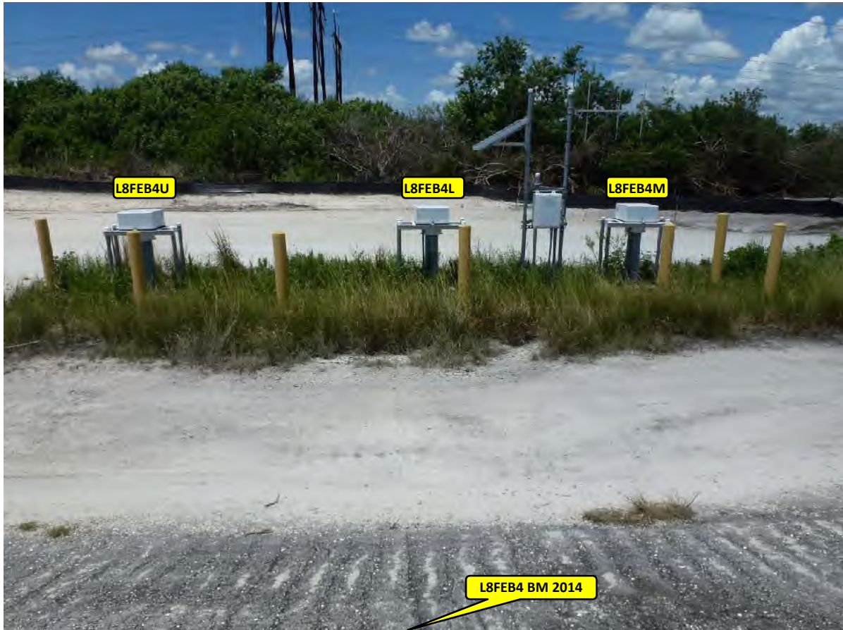
Overall Site (Looking Westerly)
