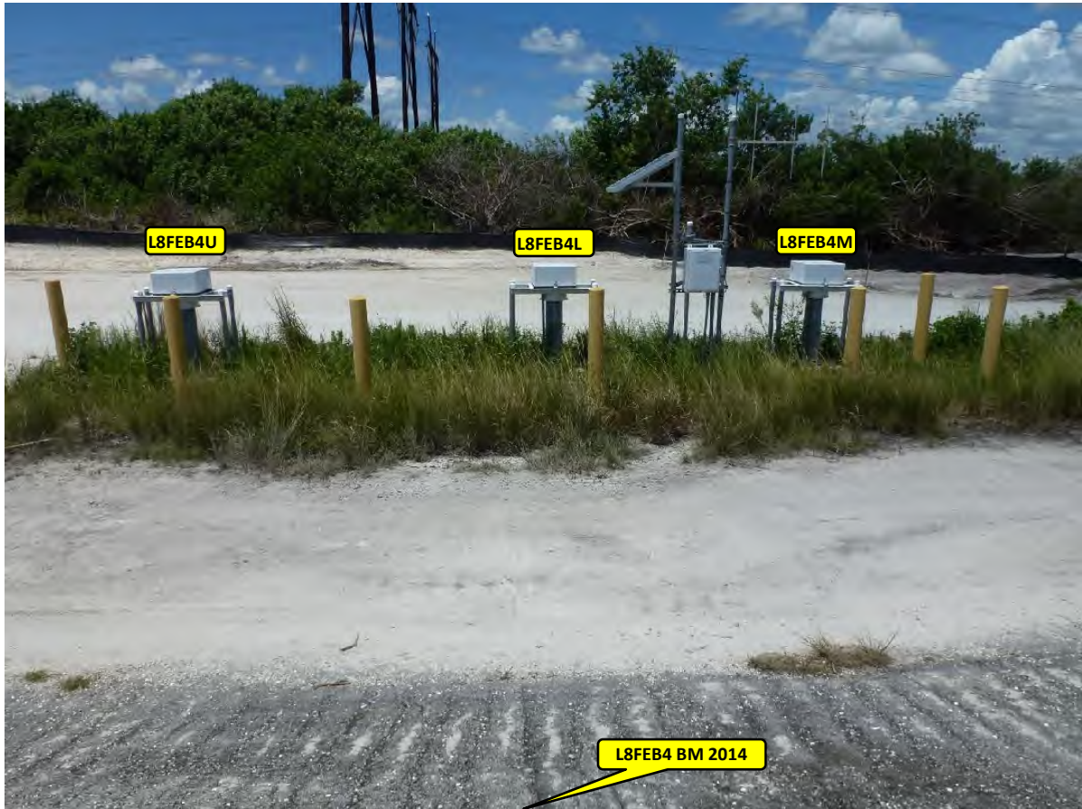
Overall Site (Looking Westerly)
