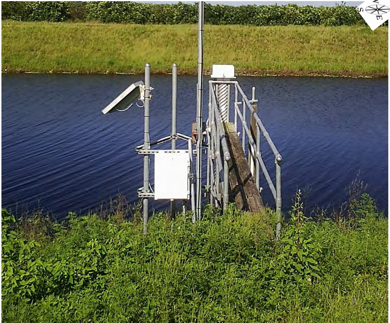
Looking Southwesterly Not to scale (photo taken 22-apr-13 by SCADA)
