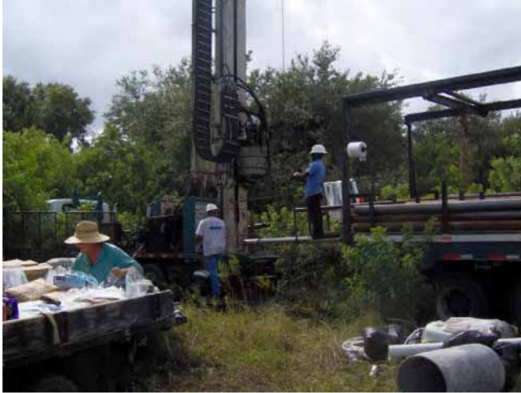
Photo 3.3 - Well Drilling at HES-29 Location
