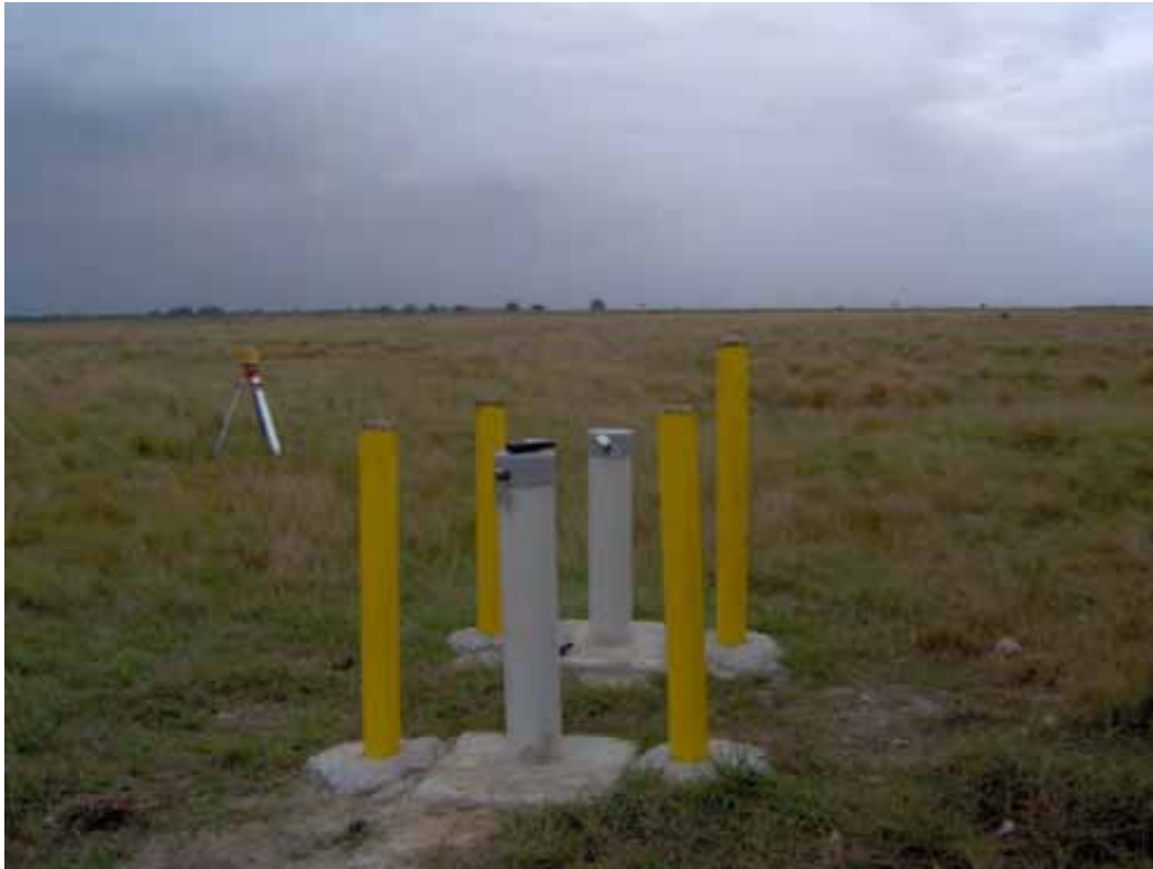
Photo 3.4 - Instrumentation of Wells HES-22 S and D
