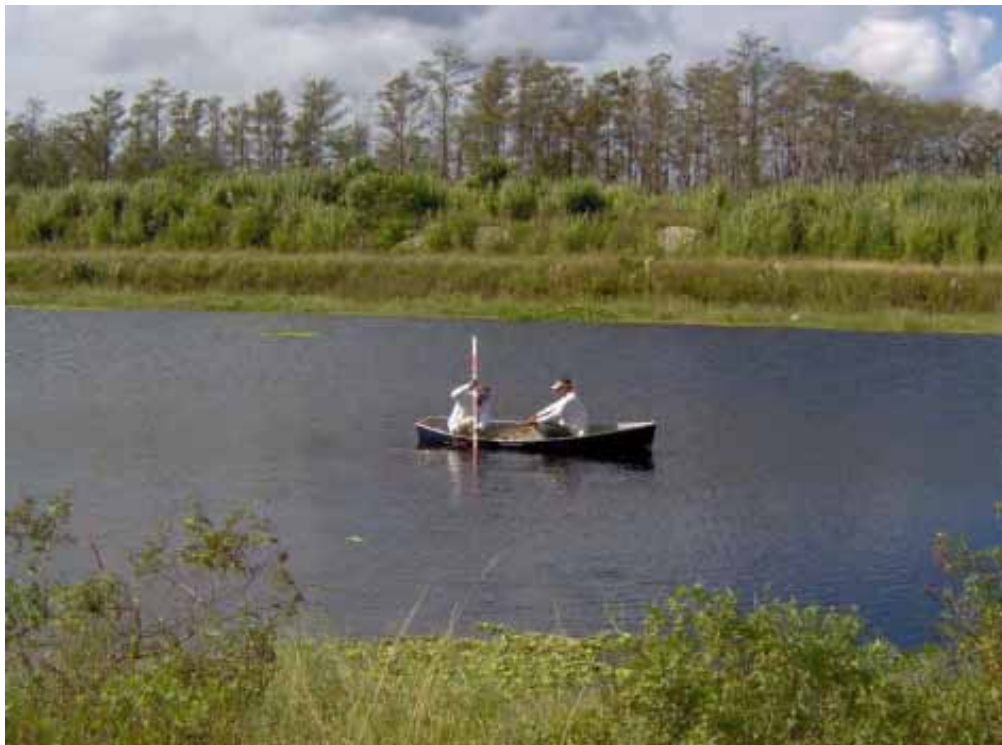
Photo 3.1 - Surveying Crew Collecting Cross Section Data in L-28 Interceptor Canal
