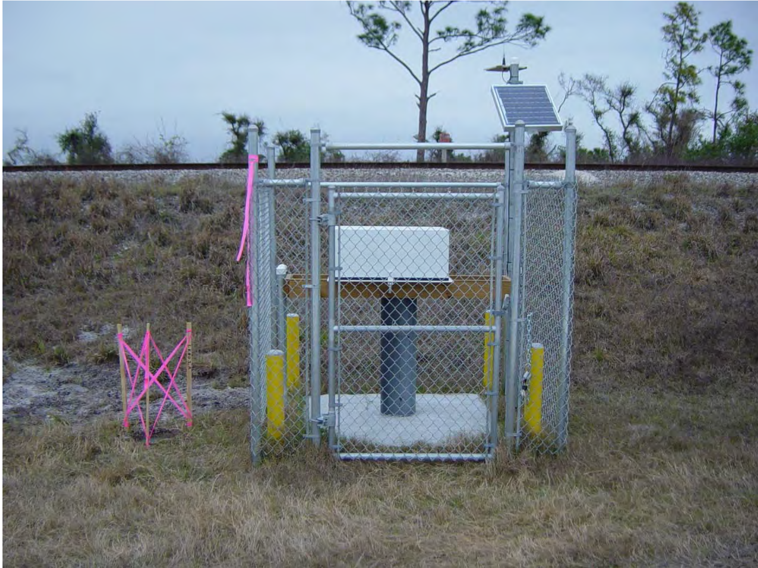
Nick Miller, Inc. Date of Photo: February 24, 2006 View: Looking at the well LKBD1A facing north
