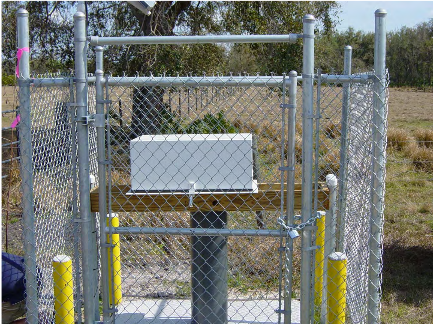
Nick Miller, Inc. Date of Photo: February 23, 2006 View: Looking at the well LKBD5C facing east
