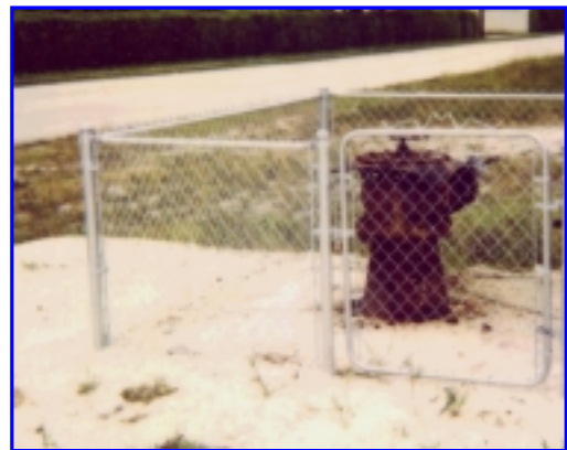
Photo 2: BF-2 (Middle Floridan Aquifer Well).
