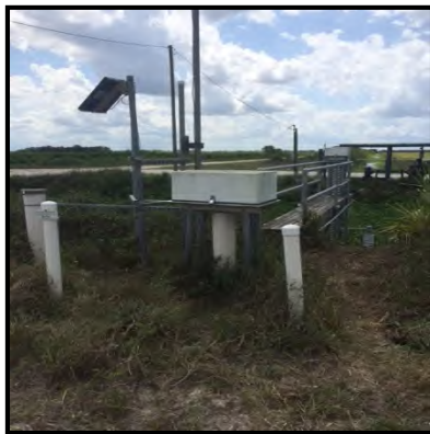
1 – Overall Site (Recorder Well, Staff Gauge, etc.)
