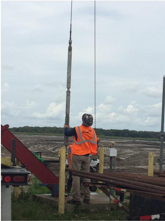
Photo 5. Installing 4-Arm Caliper Tool in Well OKF-42
