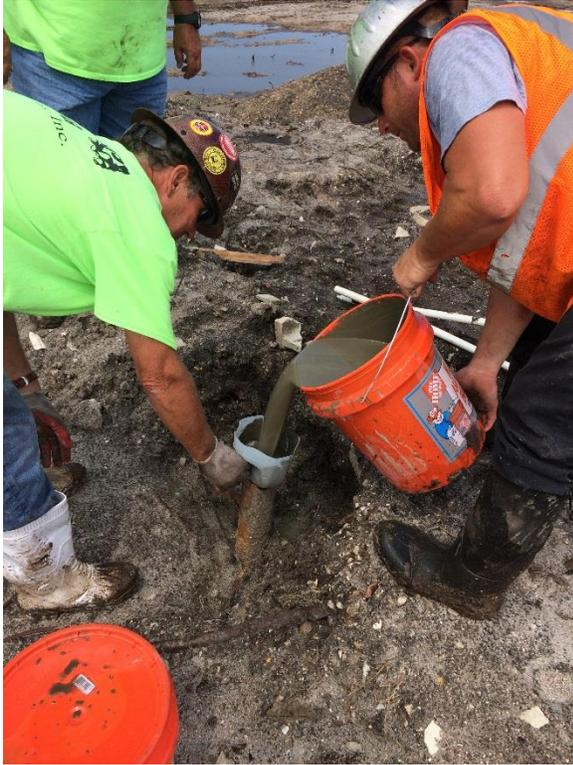
Photo 17. Placing Neat Portland Cement Grout in 3-Inch Diameter Surficial Aquifer Well
