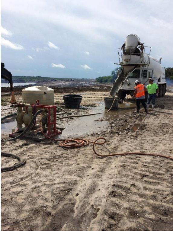
**Photo 11. Discharging Grout for Stage 2**
