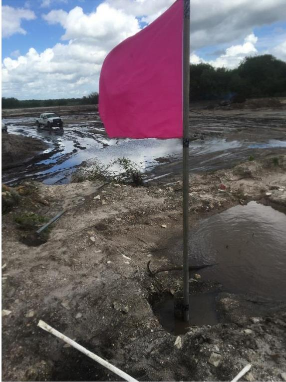
**Photo 19. Wellhead and Marker Flag at 3-Inch Diameter Surficial Aquifer Well**
