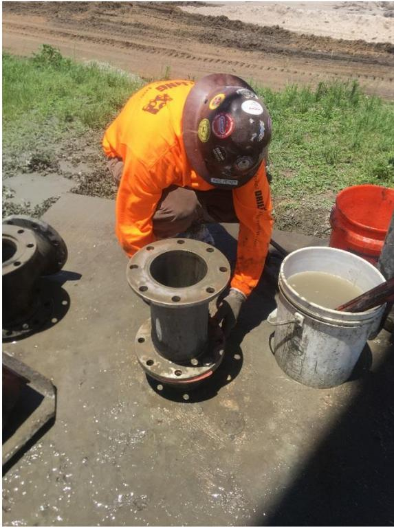
Photo 15. Dismantling OKF-42 Wellhead Following Stage 3
