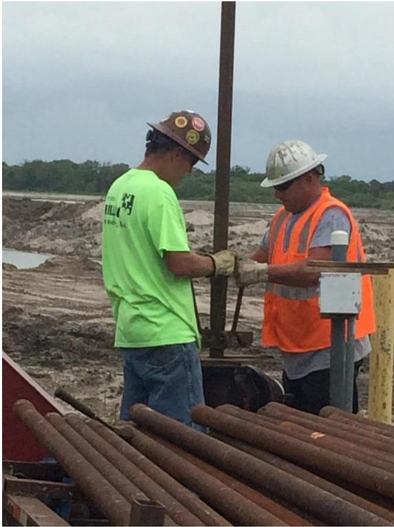
Photo 7. Setting Cementing Tubing in Well OKF-42
