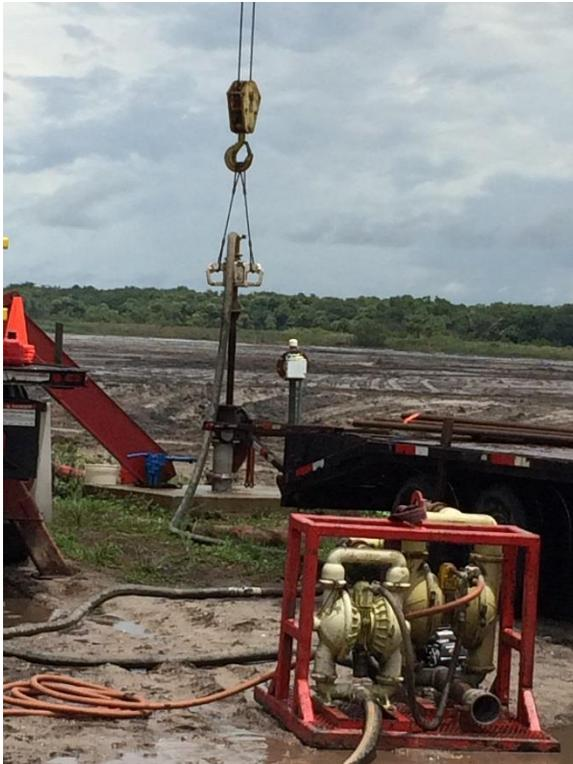
Photo 10. Cement Pump and Discharge to OKF-42 Wellhead
