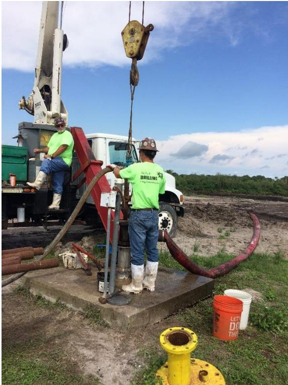
**Photo 12. Stage 2 Cementing At OKF-42 Wellhead**
