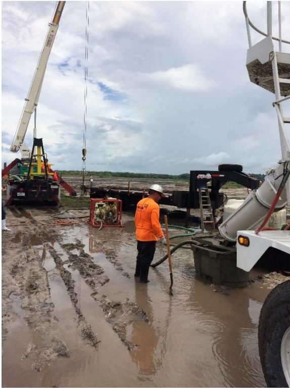
Photo 9. Discharging Grout for Stage 1
