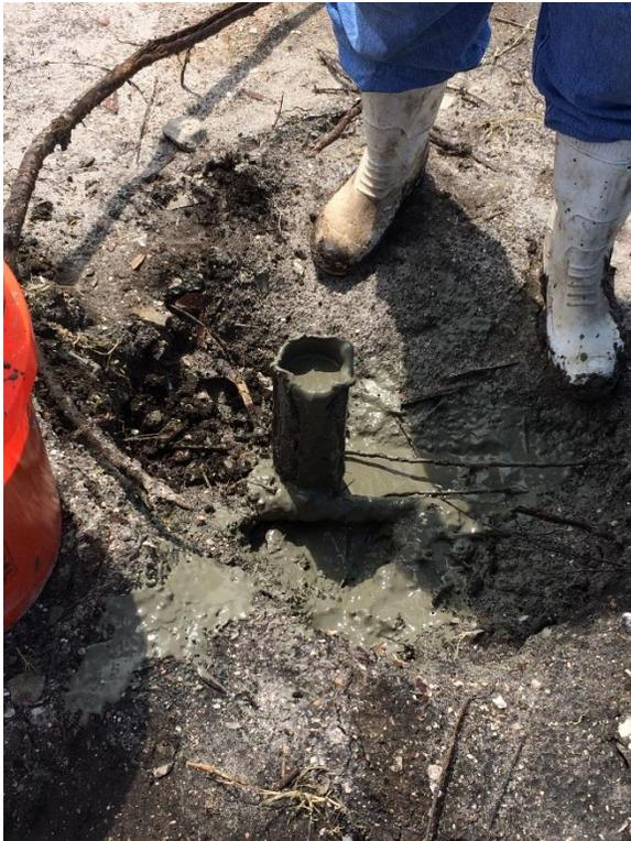
Photo 18. Cement at Completion of 3-Inch Diameter Surficial Aquifer Well Grouting
