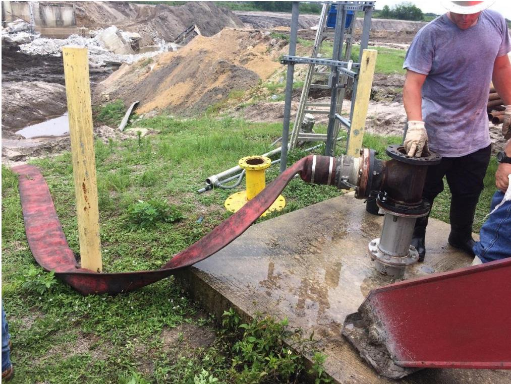
Photo 4. Discharge Line for OKF-42 Wellhead Flow
