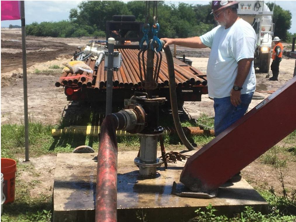
**Photo 14. Stage 3 Cementing At OKF-42 Wellhead**
