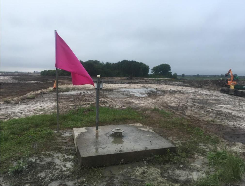
**Photo 21. OKF-42 Wellhead and Site at Completion of Well Plugging and Demobilization, 3-Inch Diameter Surficial Aquifer Well in Background (view obscured by demolition equipment)**
