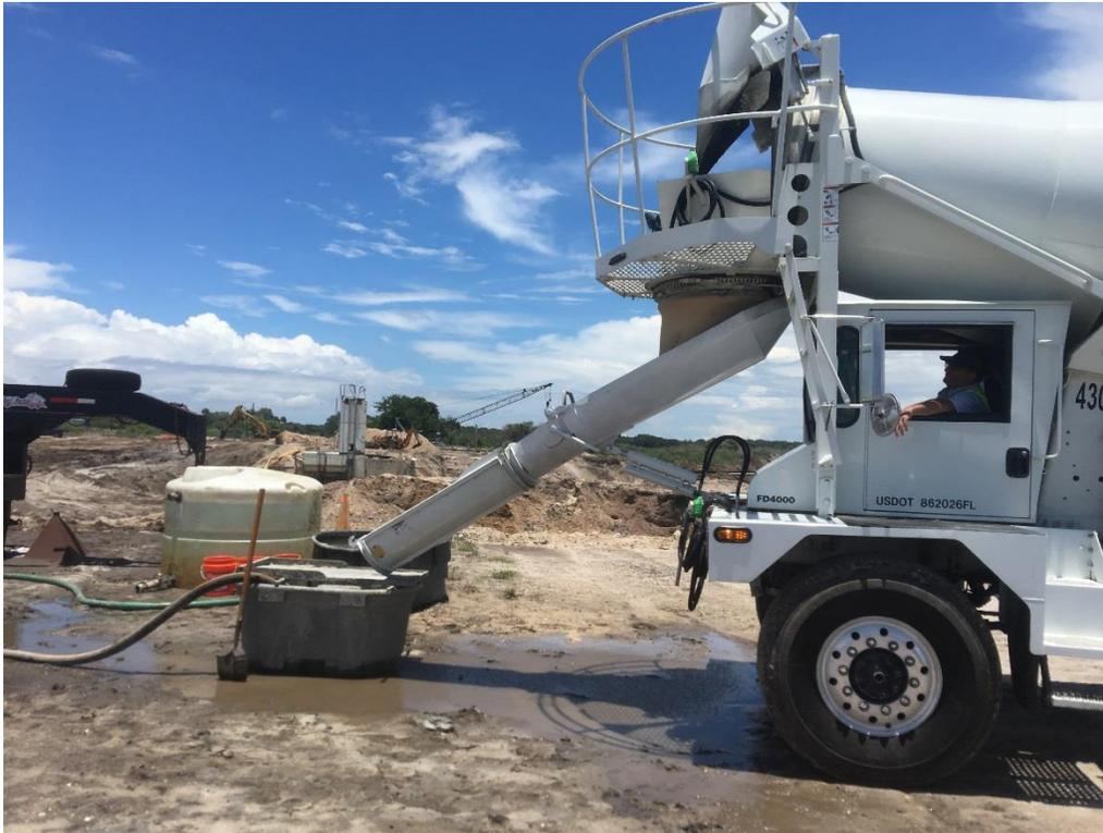
**Photo 13. Discharging Grout for Stage 3**
