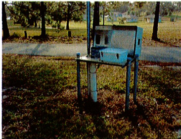
Sensor Well Area:
